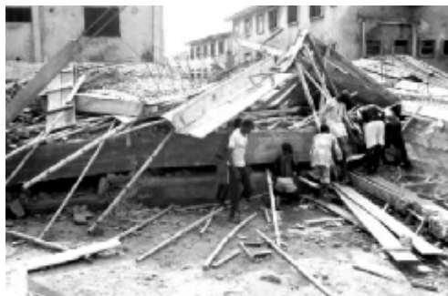
Figure 9: Remains of collapsed building (source-Leadership newspaper)
