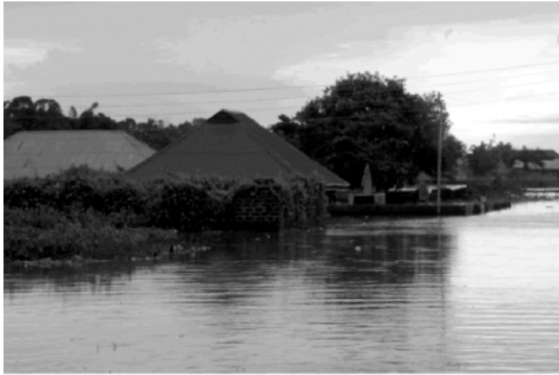
Figure 5: Flooding photos taken at Wadata in Makurdi Benue state, Nigeria (source- Photo News)
